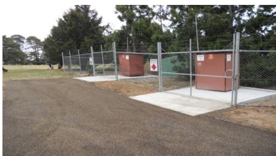
Improvements to Fuel Storage
