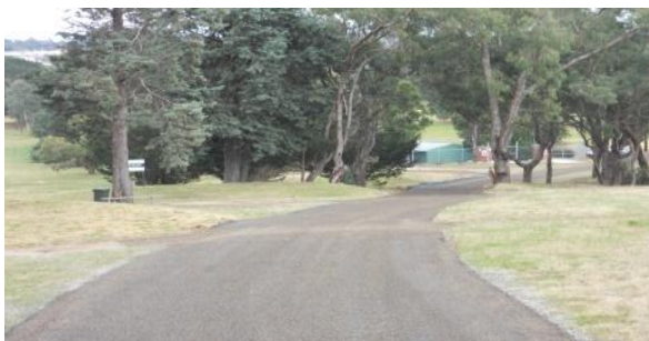
Renovated May Street Access Road
